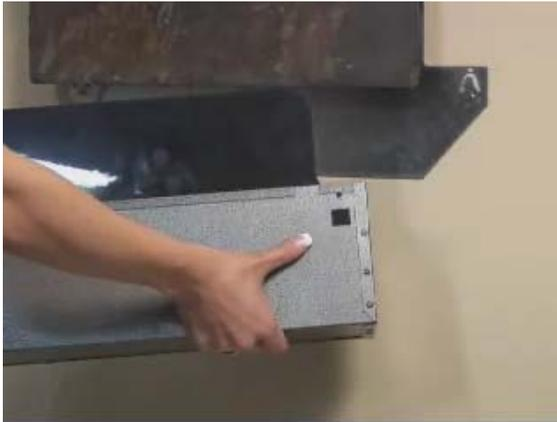
**(2) If you do not have an electrical outlet behind the stone we recommend placing the power cord behind the Water tray.** Leave approximately 6 inches of exposed cord. We can adjust the cord length later.
