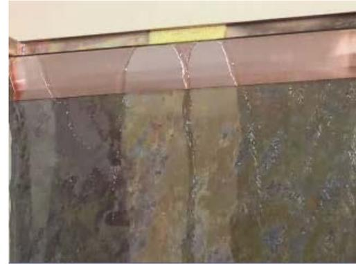
The outer edge adjusting tabs are used to control water flow at the edges of the stone. If there is a large amount of water flow at one or both edges you may experience a small amount of dripping off of these tabs. **(5) In this case, simply bend the tabs in towards the center to redirect the water onto the stone.** These tabs can also be adjusted to allow more or less water to the edge of the stone.
