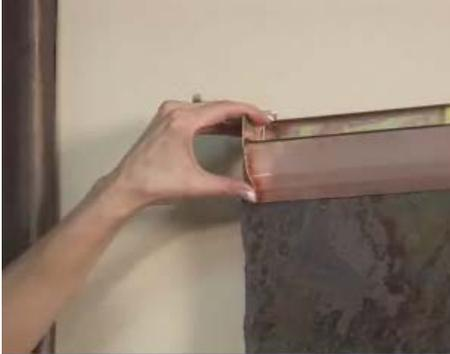
Because each installation may vary just a little **(6) your Water Distribution Unit may need to be leveled.** You can determine if it needs to be leveled by the water not flowing evenly but instead flowing stronger on one side than the other. The included leveling wedge can be used to shim either side up until it is level. The wedge
