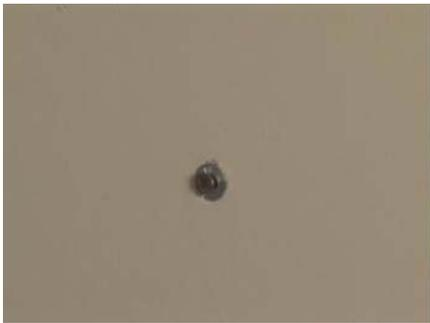
**(1) Approximately one half an inch below the dot you marked as the top center; screw an EZ anchor into the wall.** If this spot happens to be where a stud is do not insert the EZ anchor, simply screw one of the 2.5 inch grabber screws directly into the stud. Otherwise screw the 1 inch grabber into the EZ anchor. Do not tighten the screw all the way. Leave it about one quarter of an inch out from the wall.
