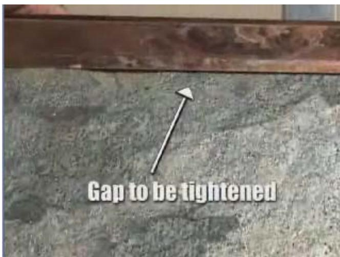
**(1) First, be sure it fits tightly on to the stone.** You can adjust the tightness using the tabs on the back of the unit.
