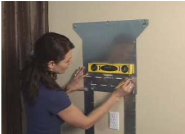
**(3) Using a carpenter's level in the lip, ensure that the bracket is level and mark all the holes including the slots with a pencil.** Once this is done remove the bracket and set it out of the way.
